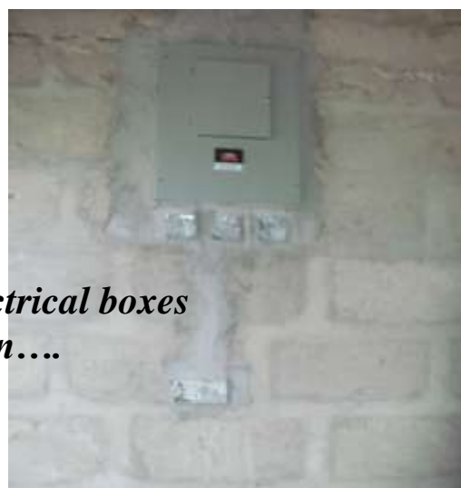
Conduit with wires running in it.
