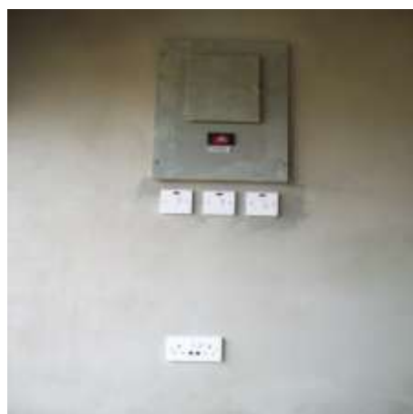
the same panel after the masons have finished their work.
